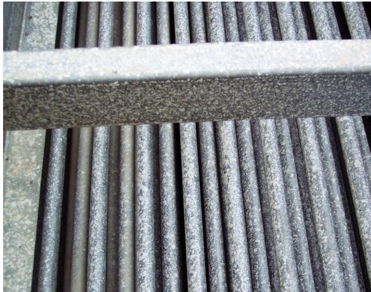
Figure 1 – Photograph of Evaporative Condenser with White Rust
